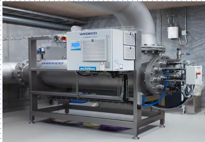
Ultraviolet water disinfection system
